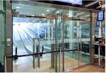
An under floor door drive enjoys a special status. The extra effort required in construction to install the drive unit below ground enables the creation of a free, airy architectural style, and therefore often plays a role in representative glass constructions.
